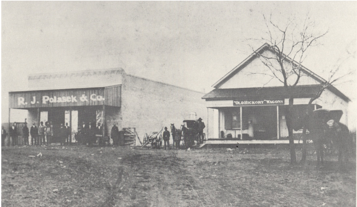
Polasek Store: Rudolph J. Polasek operated the first business in Castine in 1895, four years before the town's name was changed to Hobson. Appointed postmaster in 1898, Mr. Polasek owned a gin, lumberyard and grist mill in addition to this store. Made of brick manufactured in Hobson, parts of the wall still stand (caption and © by Karnes County Museum).
