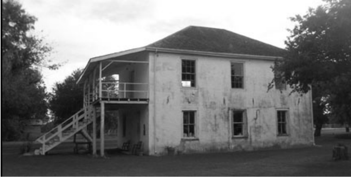
Old Karnes County Courthouse in Helena (photograph by Thomas Sajwaj, 2005)
